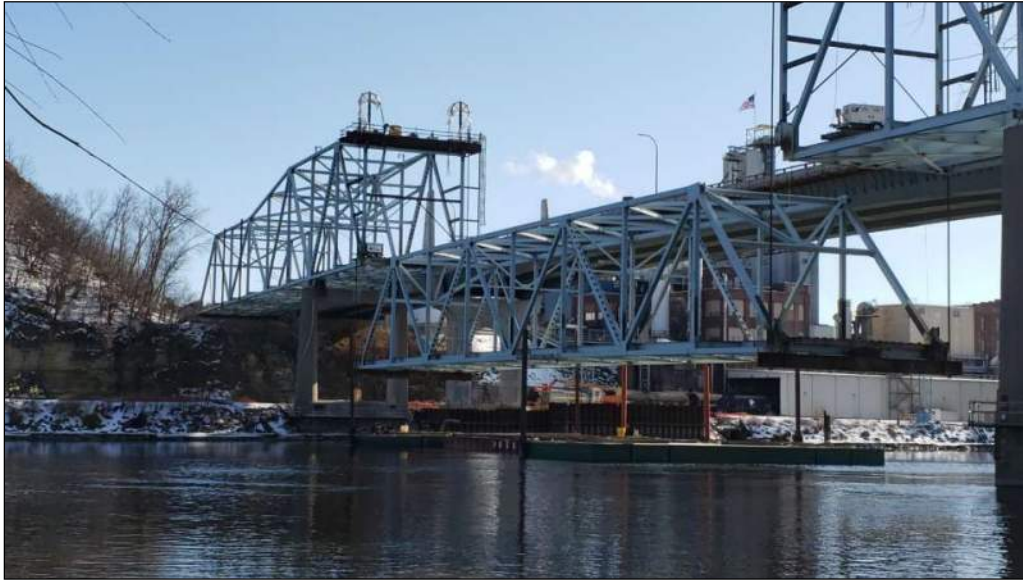
Photograph 4. Truss removal example with temporary supports and barges.
