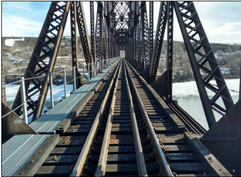
Photograph 3. Existing structure 196.6 deck.
