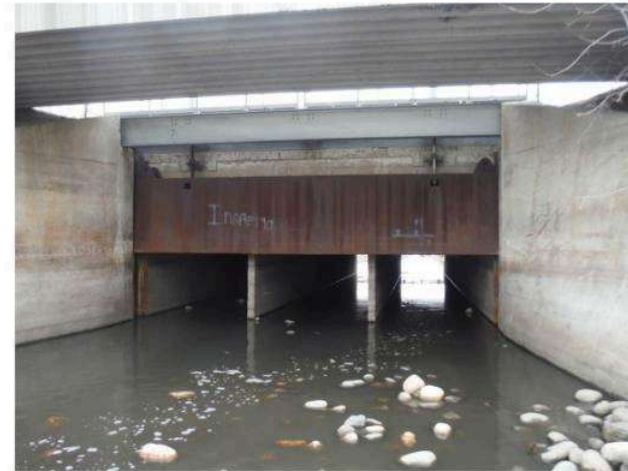
View Looking East
